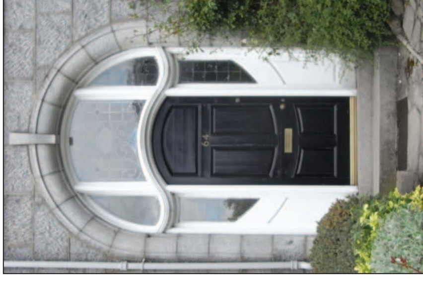
Windows, doors and doorways can be important features of a building which are important to protect
